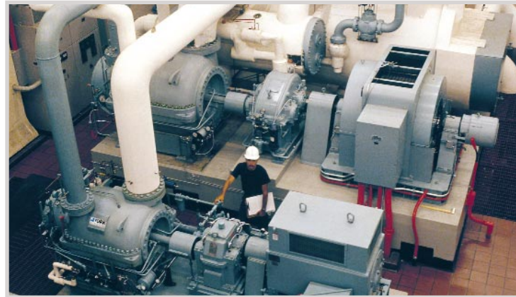
The versatility of the Titan chiller is evident in this parallel-drive installation.
