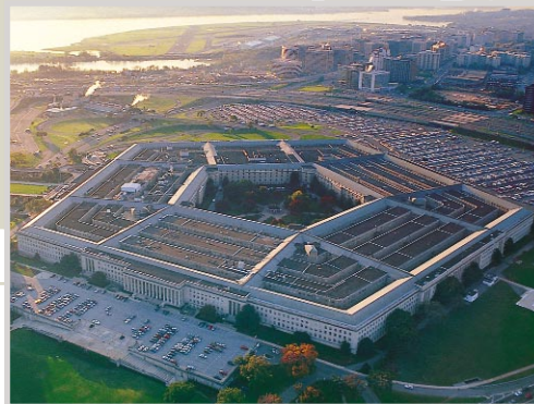
At 6.6 million square feet (610,000 square meters), the United States Pentagon is one of the world's largest office spaces, requiring 37,500 TR (132,000 kW) of cooling by Titan chillers.
