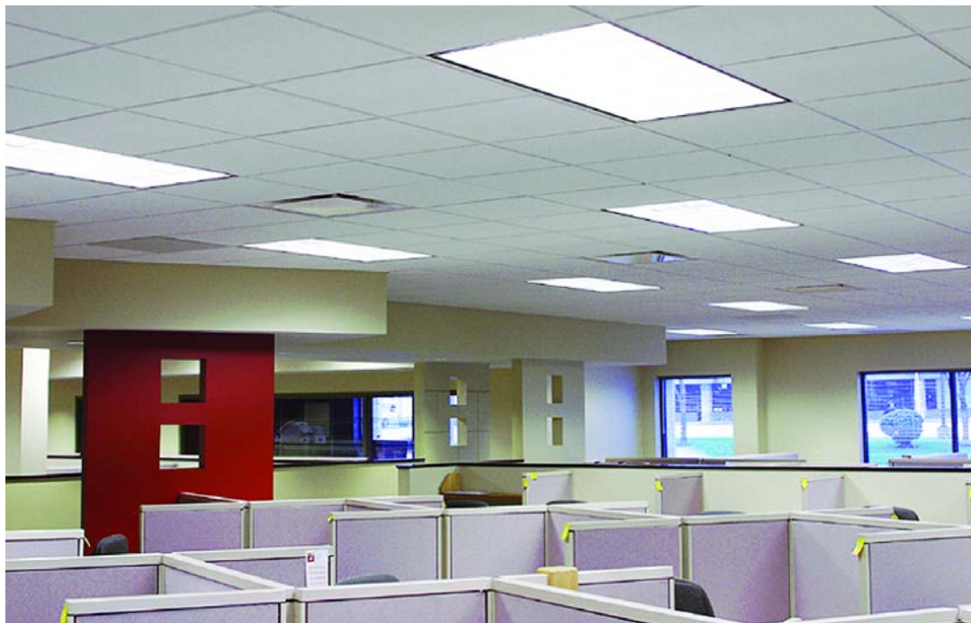
Finished construction is the familiar drop-ceiling design.
