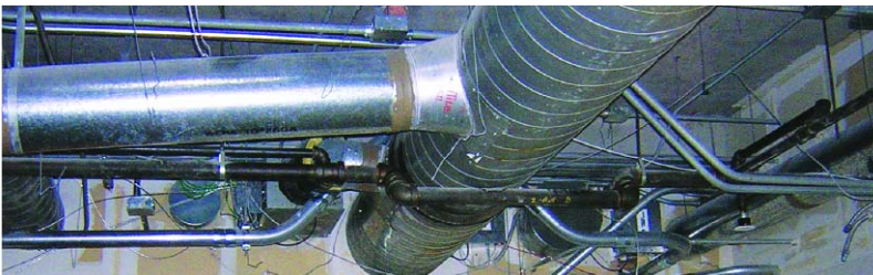
Typical congestion found in an overhead air-distribution system using ductwork
