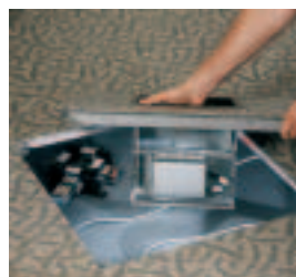
MIT Variable Air Volume Unit (with Plug and Play Cable Management)
