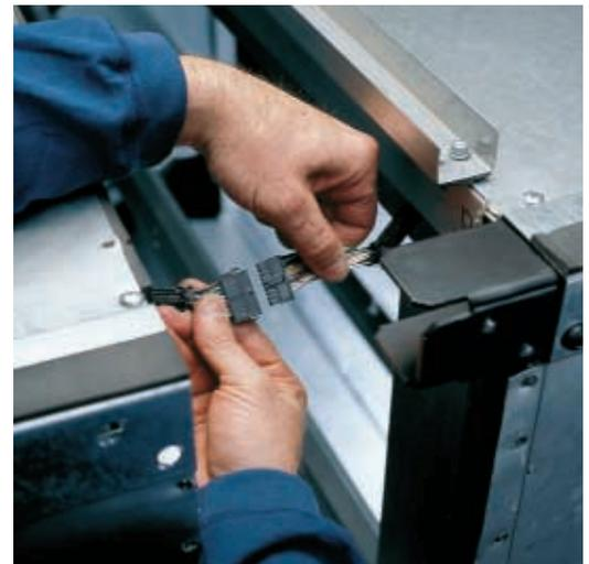
In some instances, the AHU is too large to ship in one piece, and must be split. To ensure fast and easy jobsite assembly of the OptiLogic controls, labeled quick-connects come standard on all shipping splits.
